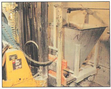
Mixing ingredients into a mobile hopper
